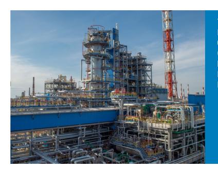
THE LIST OF MAJOR PROCESSES COMPRISES: PRIMARY PROCESSING OF OIL AND STABLE GAS CONDENSATE, CATALYTIC CRACKING, CATALYTIC REFORMING, DIESEL FUEL HYDROTREATMENT, AROMATICS PRODUCTION, FUEL OIL AND BITUMEN PRODUCTION ETC.
